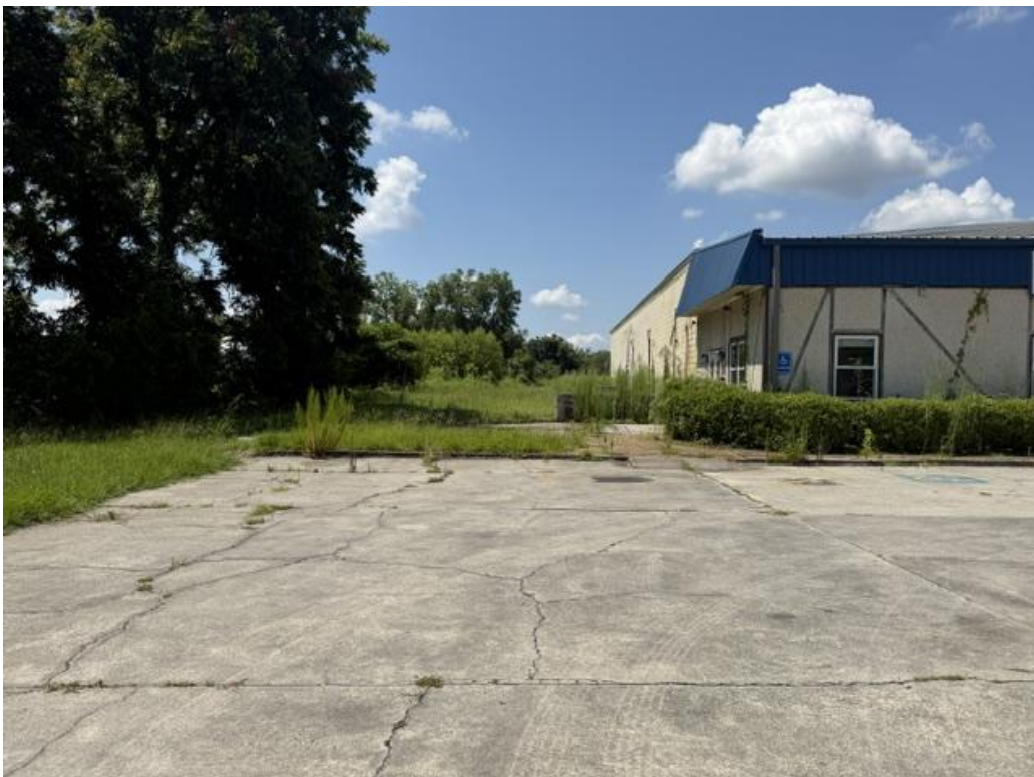
Subject property: view of the east side property from the ROW on Johnson Street, facing south.
